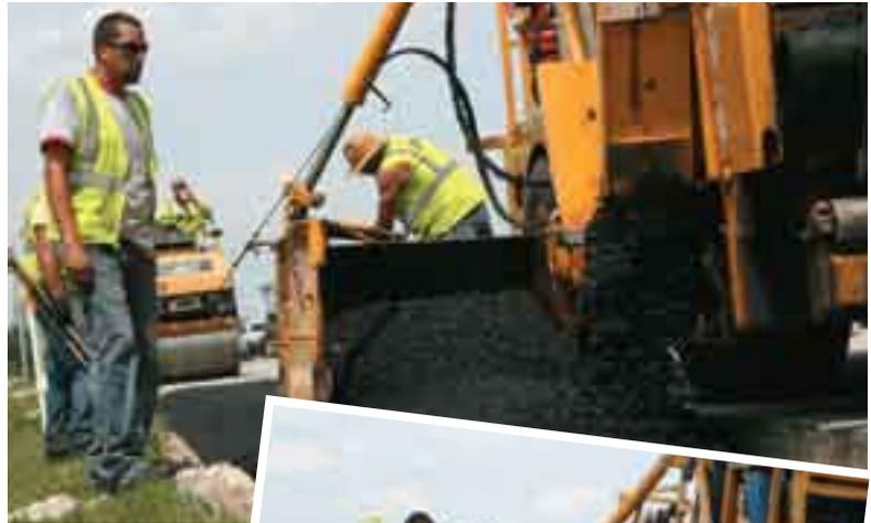
Gallagher Asphalt's road widener paves the first lift of a 6-inch base course of warm mix on Route 53's shoulders
