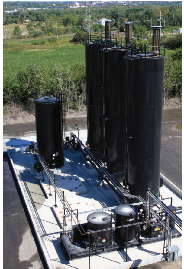
The plant includes a new tank farm with concrete secondary containment for the three 35,000-gallon liquid asphalt storage tanks.
