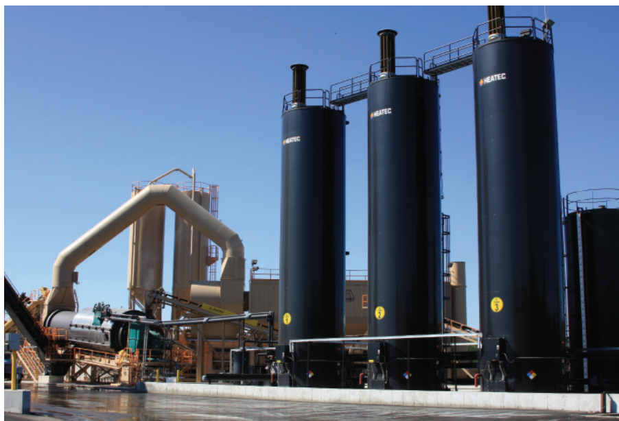
Struggling to keep up with product demand, Gallagher upgraded its Joliet facility to a 500-tph Astec Double Barrel plant.
