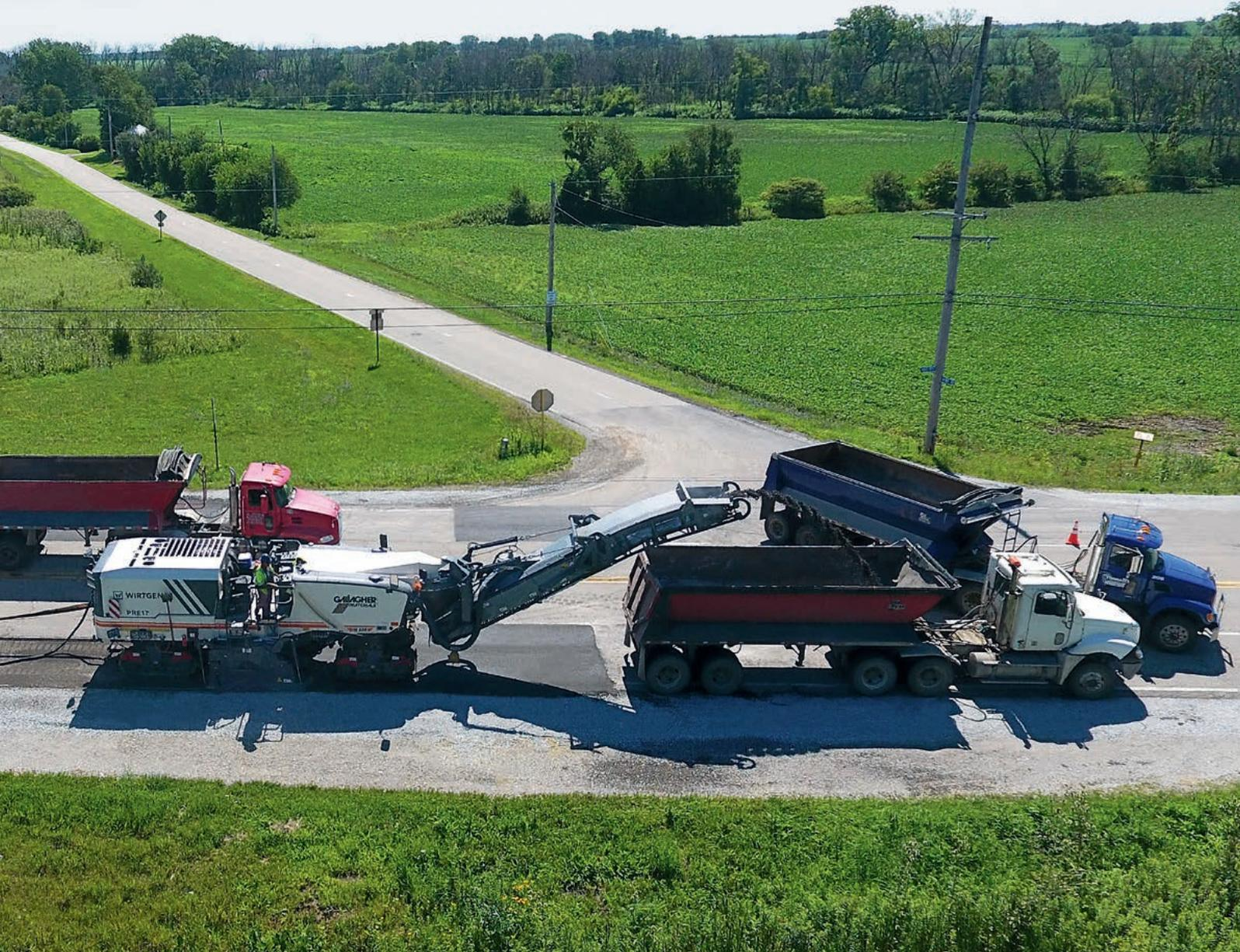
cold milling machines are extremely versatile to use, covering everything from standard applications through fine milling for the creation of new, level road surfaces to the use of what are known as ECO cutters for a particularly high area performance. This increases the capacity utilization of the large milling machine, boosting its economic efficiency in the process.
